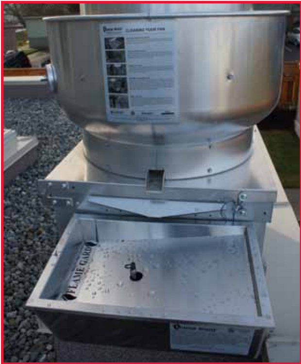
Model EFI-UB shown installed on fan
